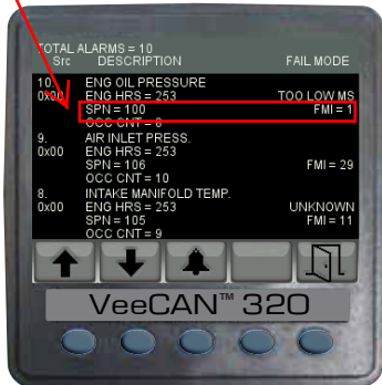
Alarm Screen after Alarm Acknowledge
